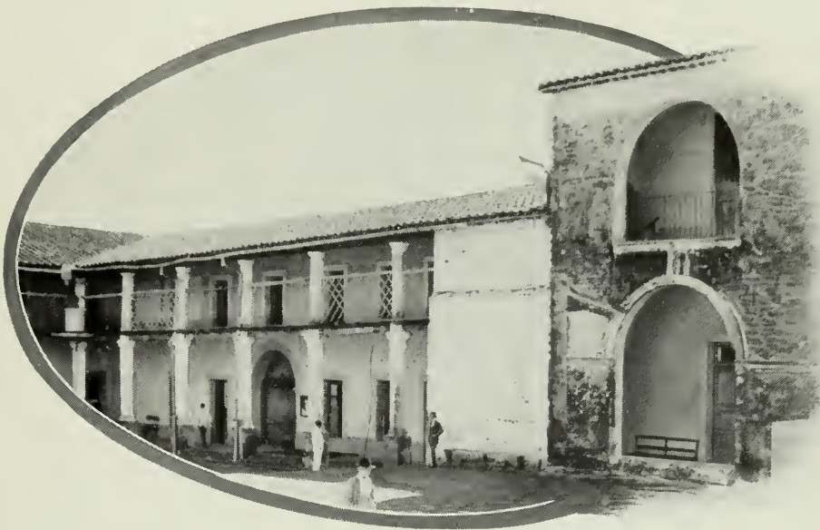
HOUSE IN ASUNCION ONCE OCCUPIED BY MADAM LYNCH, NOW USED AS BARRACKS.
